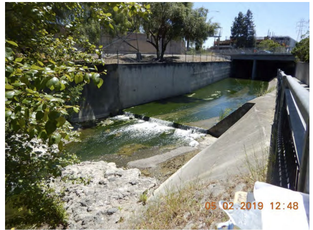
Photograph 3: Highway 101 culvert and chute
