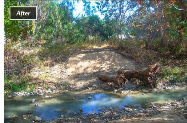
Looking perpendicular to channel after large woody debris installation.
